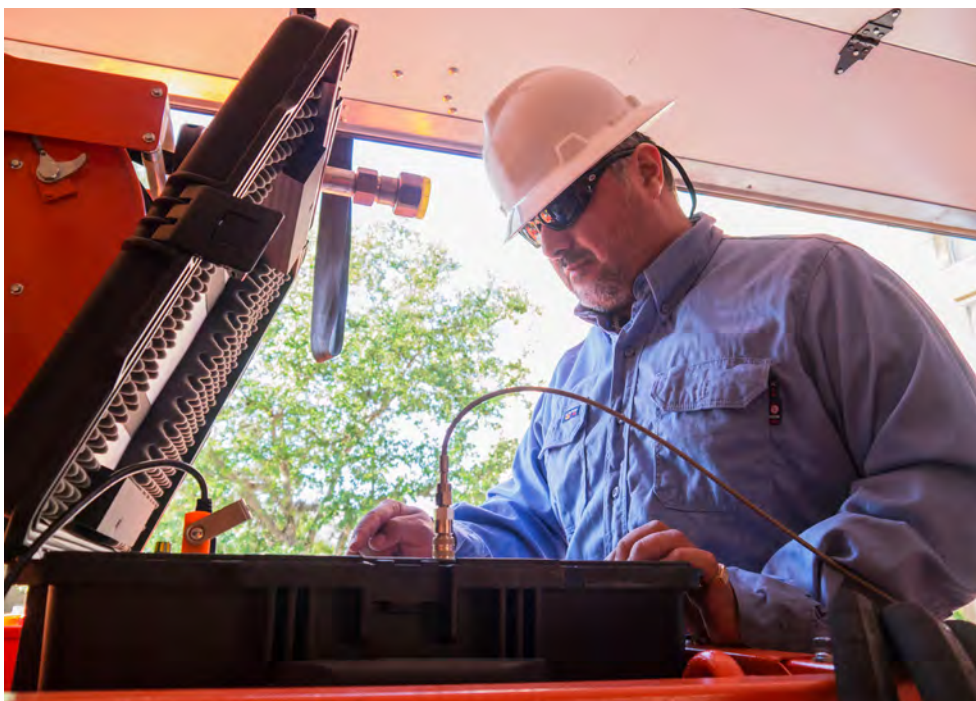
Figure 2: Analysis equipment measures purity and contamination levels in SF 6 gas
